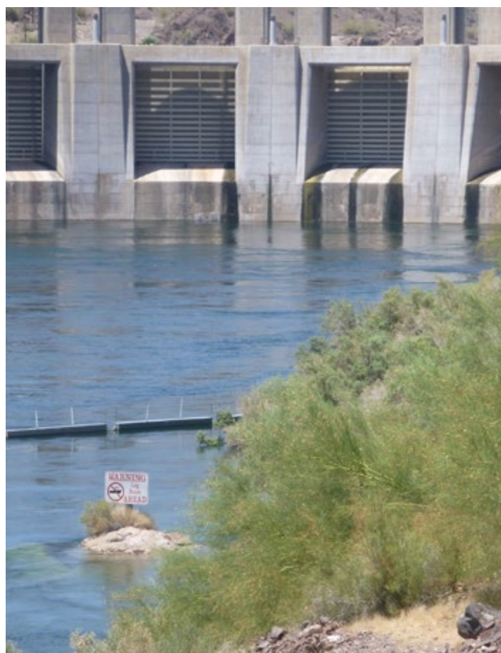
Tailrace of Parker Dam
